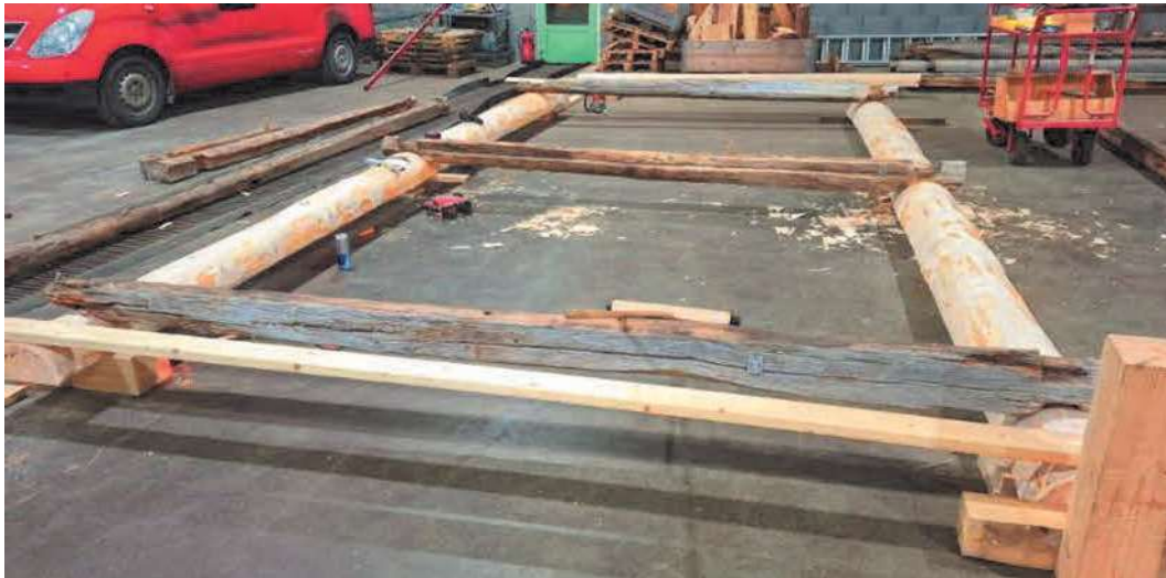
Figur4. nye sviller under montering
